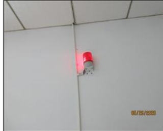
External photo(s) of the production unit(s) Fire alarm testing onsite.jpg
