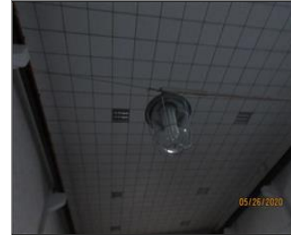
External photo(s) of the production unit(s) Anti-explosive light.jpg
